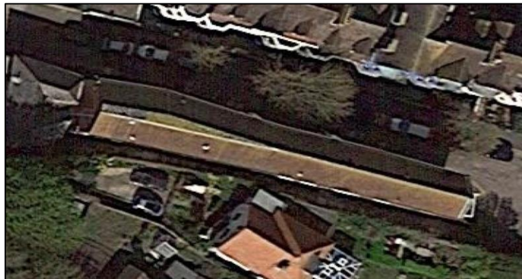
Fig.2: Flat roof area visible to left end of building.
