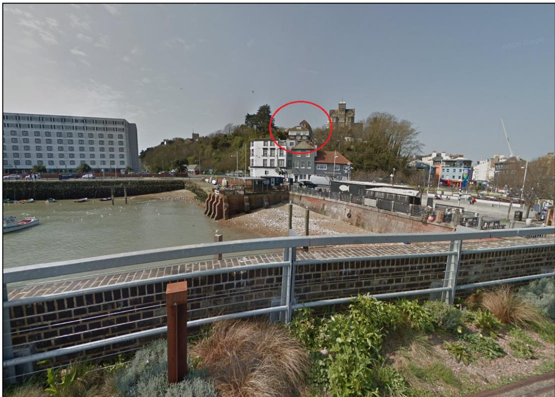
Fig.11: View from the harbour bridge, roof of Bayle Court circled
